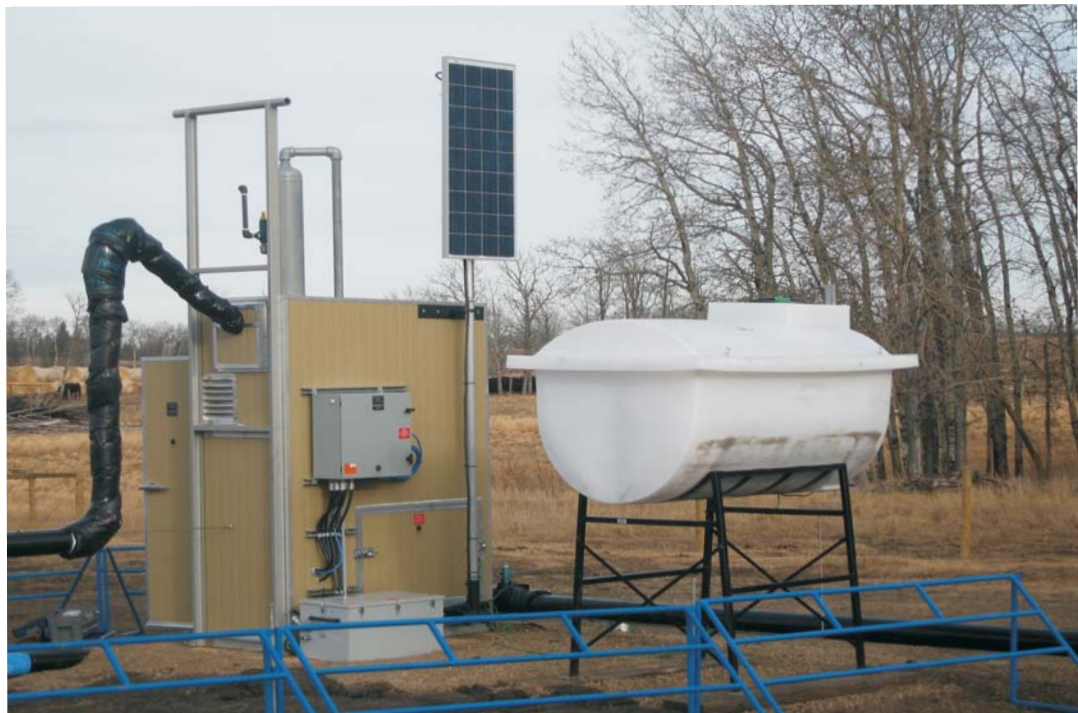
Central Alberta Installation with our Bear Cyclone Separator
