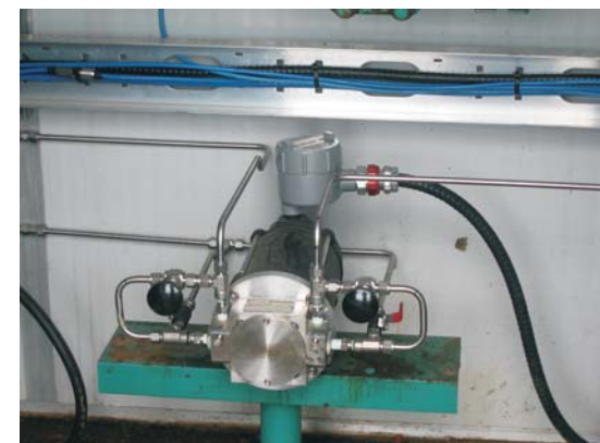
Electric Chemical Pump
