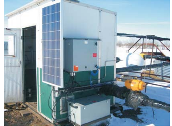
Bear Controller Retrofit
