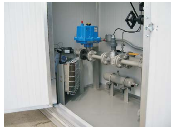
Electric Actuator
